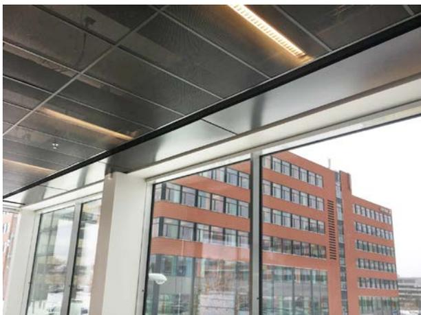
Radiant heaters are the perfect protection against cold draughts. Here the windows are protected by suspended Aquaztrip Plan with black finish.
